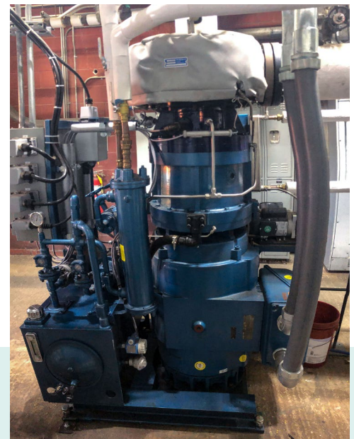
▲ A plug-and-play, skid-mounted turbine that is easily piped into existing steam systems.
